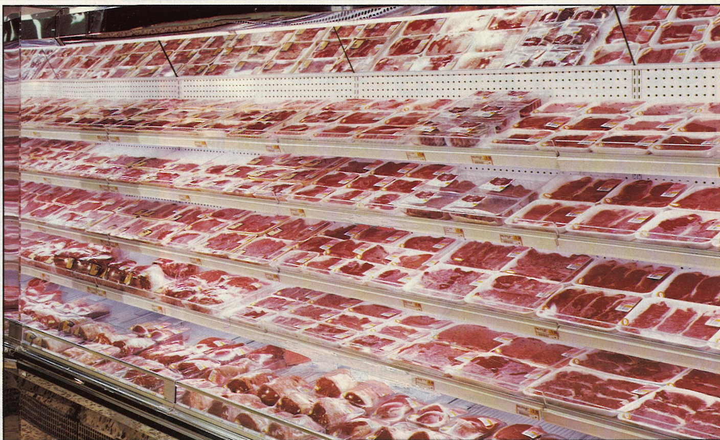
A multi undershelf lighting system in a refrigeration cabinet producing good colour rendering.
